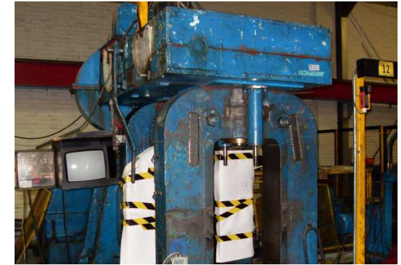
Damaged press after metal stitching repair
