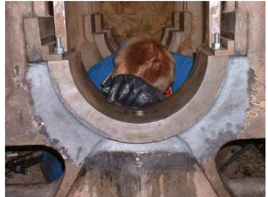
Replacement of A Main Bearing Pocket
