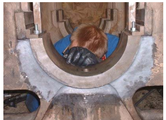
Finished Repair After Hand Dressing
